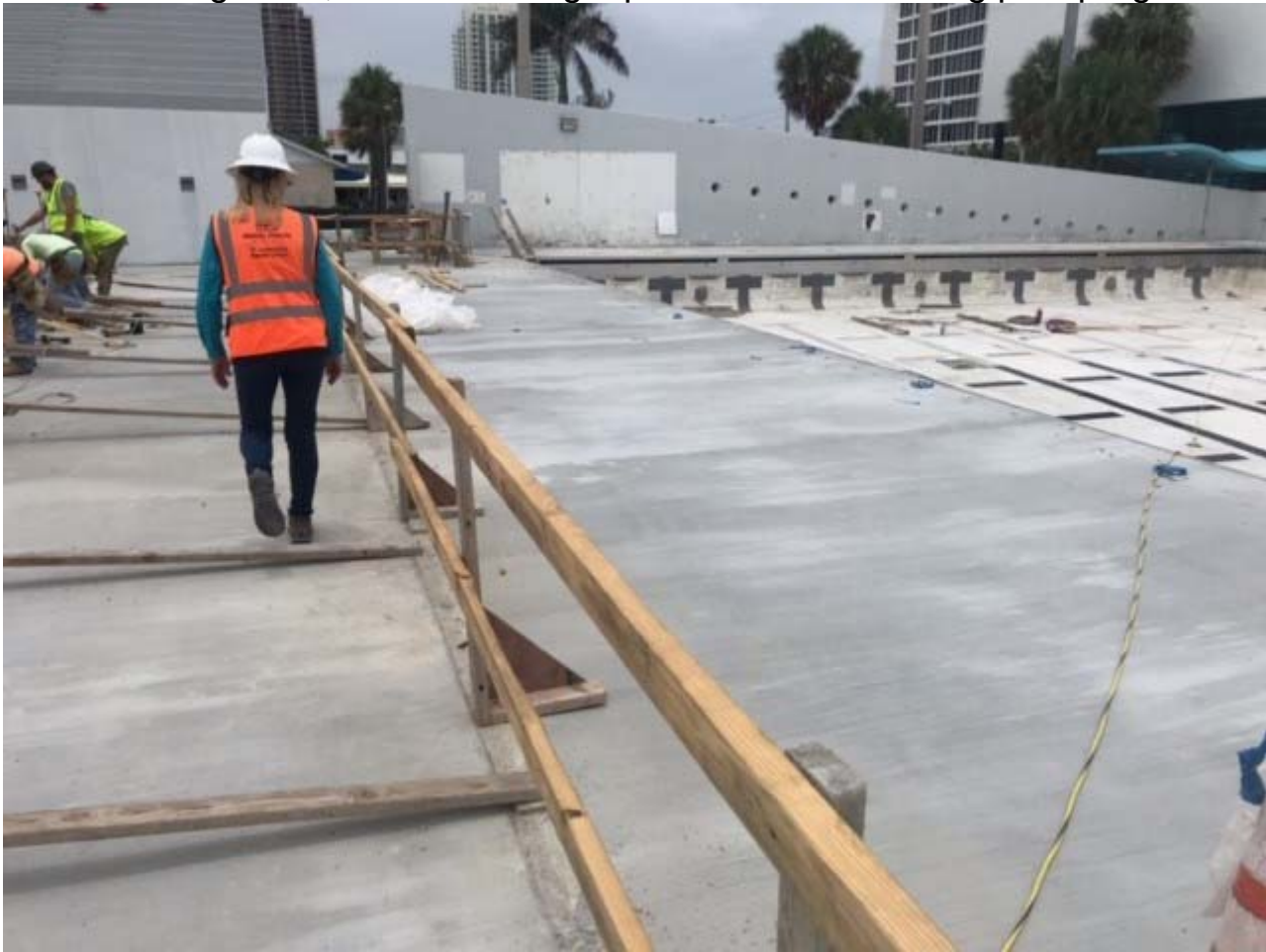
This guardrail is mid point between the training and competition pools. The piece of plywood strip at the base of the fence protects the deck drain from debris during construction.
