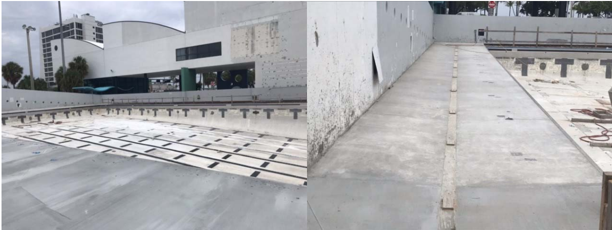
This guardrail is mid point between the training and competition pools. The piece of plywood strip at the base of the fence protects the deck drain from debris during construction.
